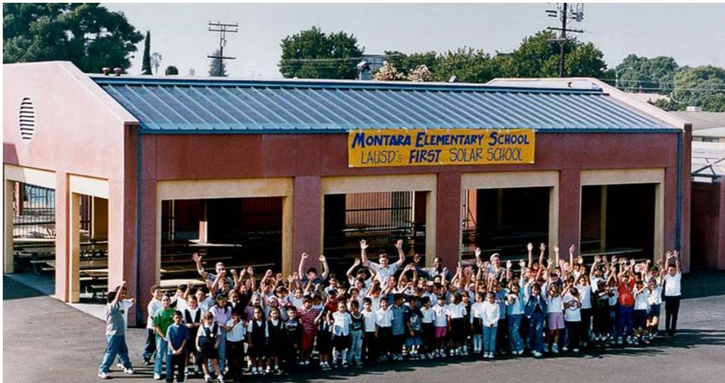
Montara Elementary School lunch room with BIPV on the roof
