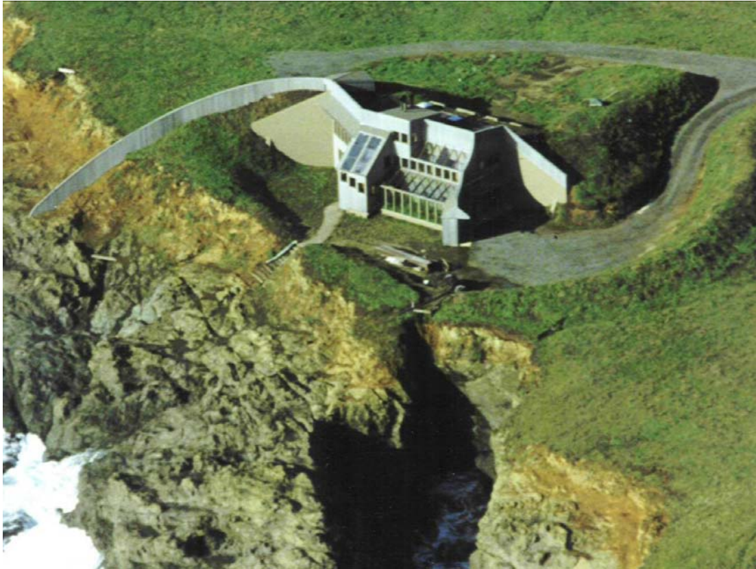
View from the South/East
