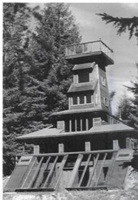
A solar home featuring integrated photovoltaics and solar water heaters as well as a solar radiant floor.
