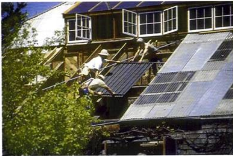
Workers install a roof-integrated solar hot water panel. Top Right: Sonoma State energy major graduates help install an integrated photovoltaics array.
