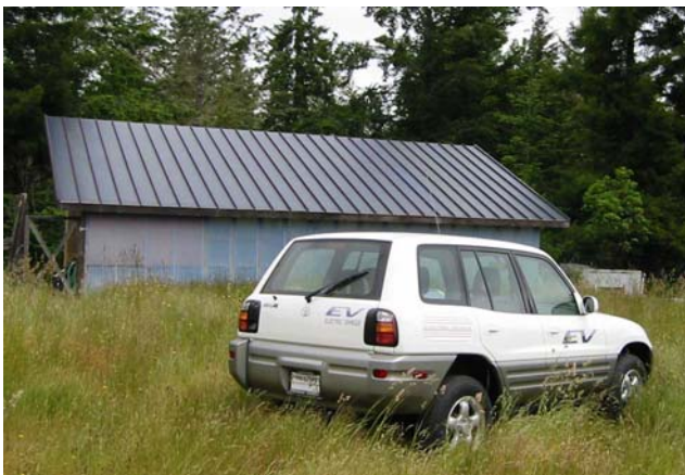
Our E-RAV and PV charging station
